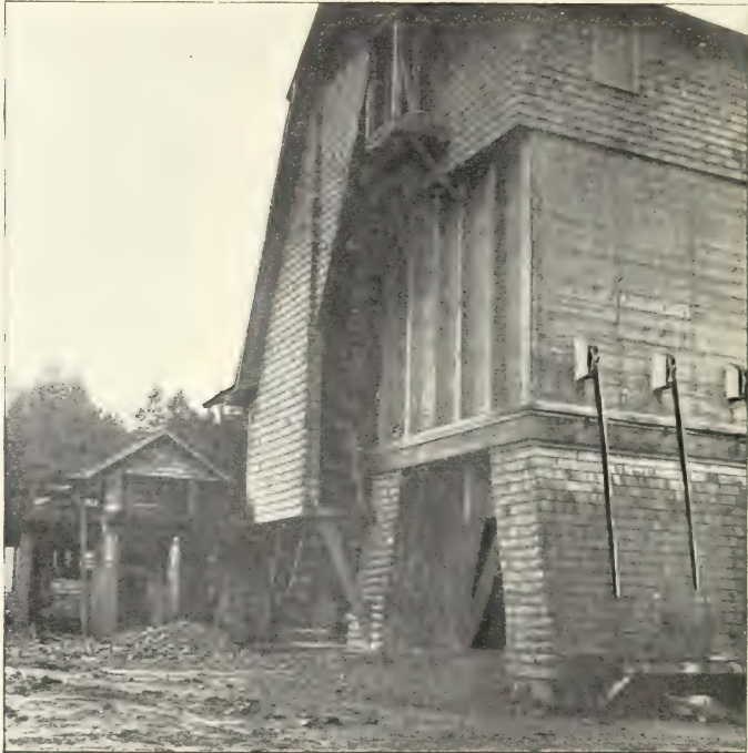
Where Stone is Loaded. Each Lever as it is removed gives a different size stone
